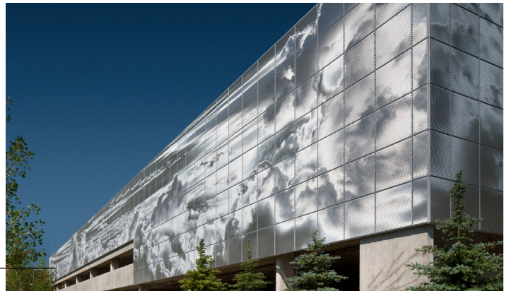
SAIT Parking Garage Calgary, Canada
